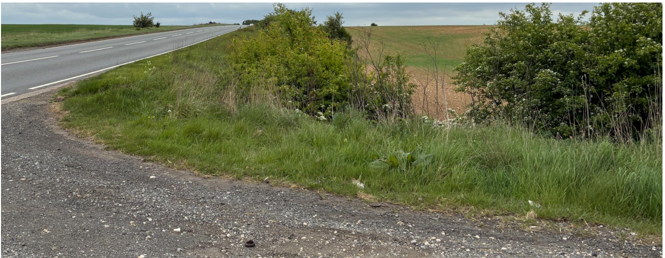
Gorse Hill Lane: Significant levels difference between existing carriageway and adjacent field
